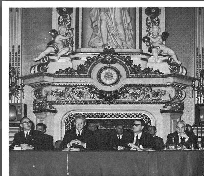
Partial view of the table of honour during the ceremony. In the foreground, from left to right, can be seen Mr. C. J. Griffiths, Mr. Maurice Couve de Murville, Mr. Jacques Marette and Mr. Gerald C. Gross. (Ministry of Posts and Telecommunications, Paris)
