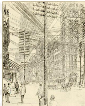
Etching of Overhead Telephone and Telegraph Wires in Broadway, 1890 Book of Old New York Henry Collins Brown 1913
