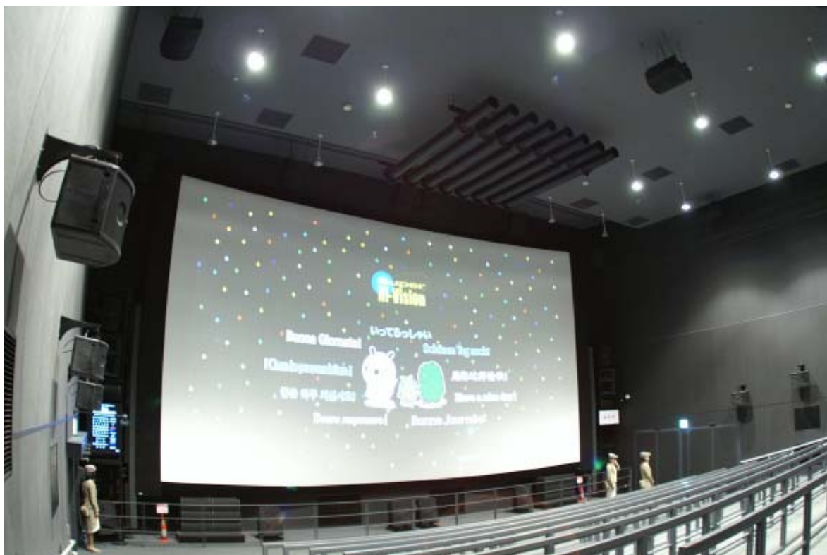
FIGURE 3 Theatrical 22.2 multichannel sound system at World Exposition held at Aichi, Japan in 2005
