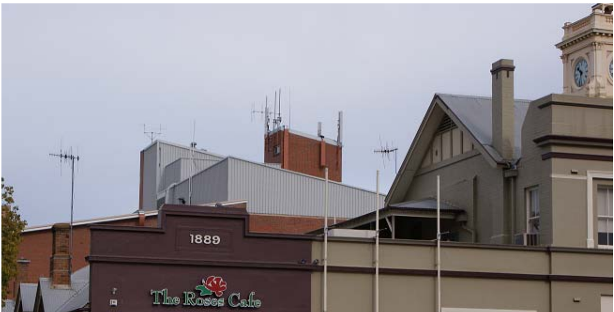
FIGURE 31 Base station at Goulburn city centre
