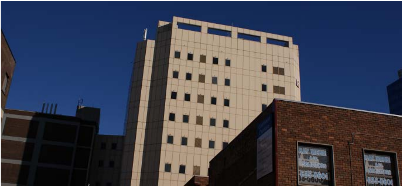
Base station at Marsden Street, Parramatta
