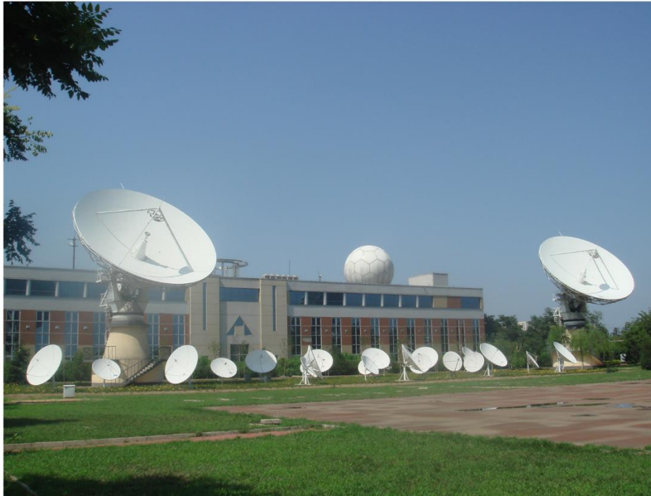
FIGURE 6 TVRO antennas for broadcast monitoring
