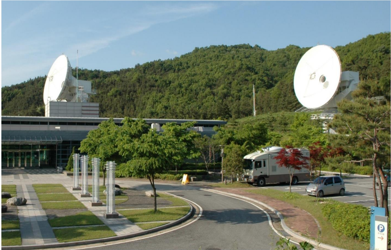
FIGURE 7 Antenna 1, 2 in SRMC
