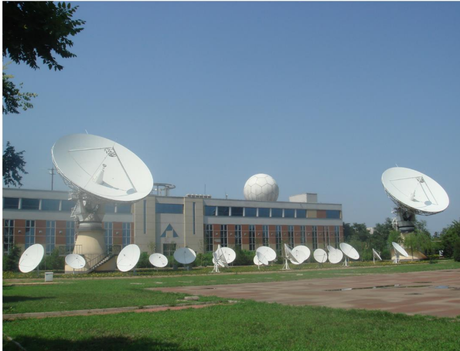
FIGURE 6 TVRO antennas for broadcast monitoring
