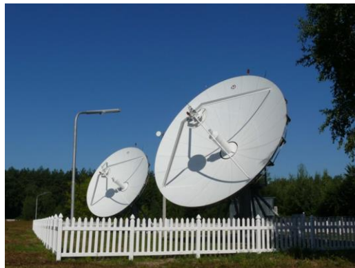
UCRF satellite monitoring station antenna system
