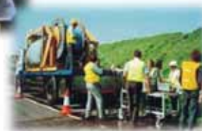
Floating techniques for installation of fibre-optic cables
