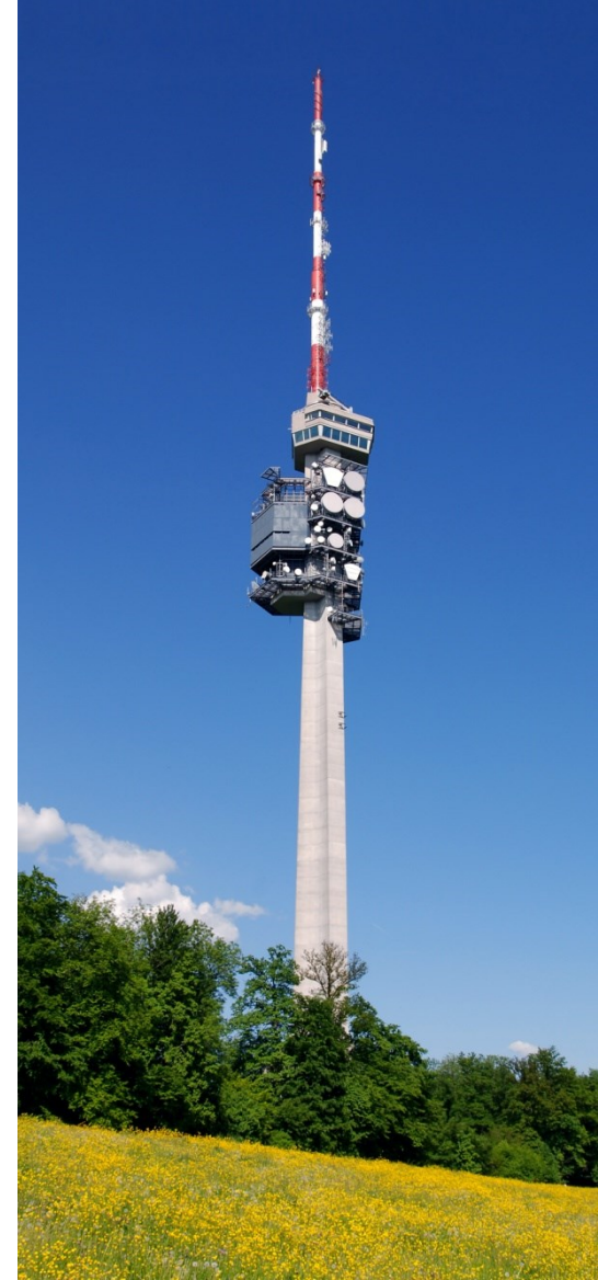
Television Tower St. Chrischona, Switzerland Source : wikipedia
