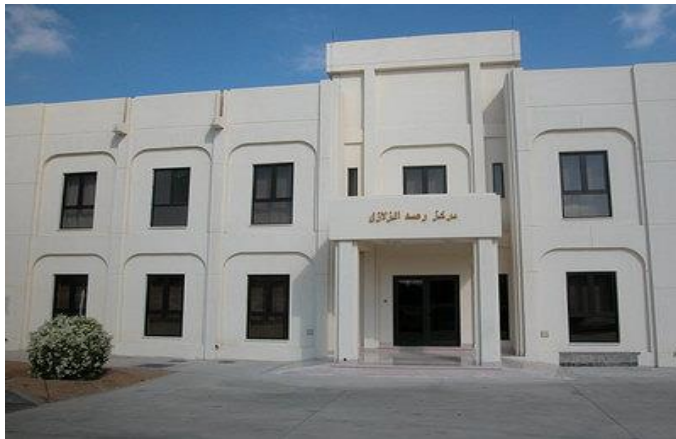
Earthquake Monitoring Center @ Sultan Qaboos University
