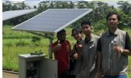
Solar Power Integration
