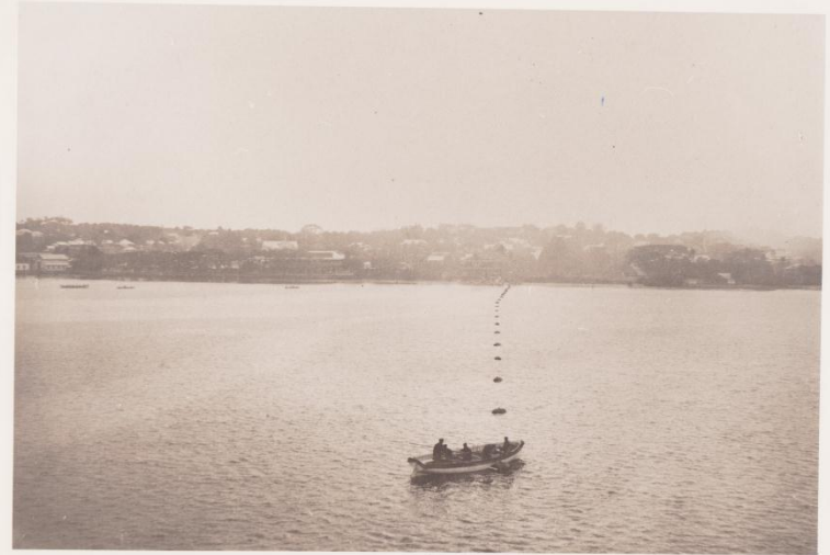
CABLE SHORE END LANDING - 1902
