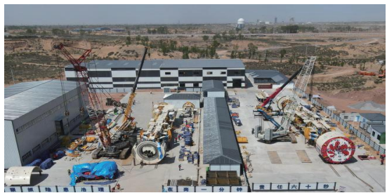
5G+Large equipment assembly
