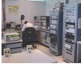
Electrical and RF
