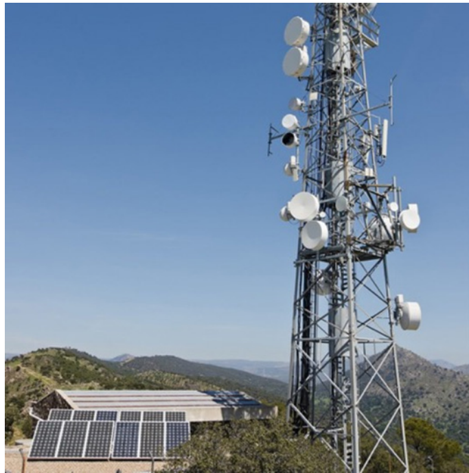
Figure 34: ESCO power solutions in Africa
