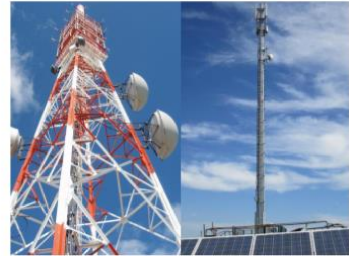
Fig. 1. Antennas mounted on a lattice tower (on the left), antennas mounted on a monopole (on the right).
