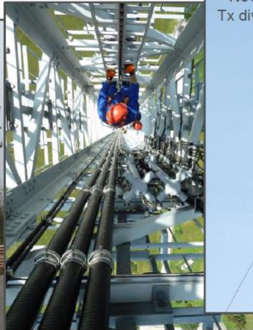
370 m of RF-cable 4" installed in one run
