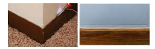
Invisible optical cables can be used for indoor wiring. The invisible optical cable is a kind of transparent sheathed optical cable, which can be pasted on the surface of the indoor wall through a hot melt glue gun to complete the laying.
