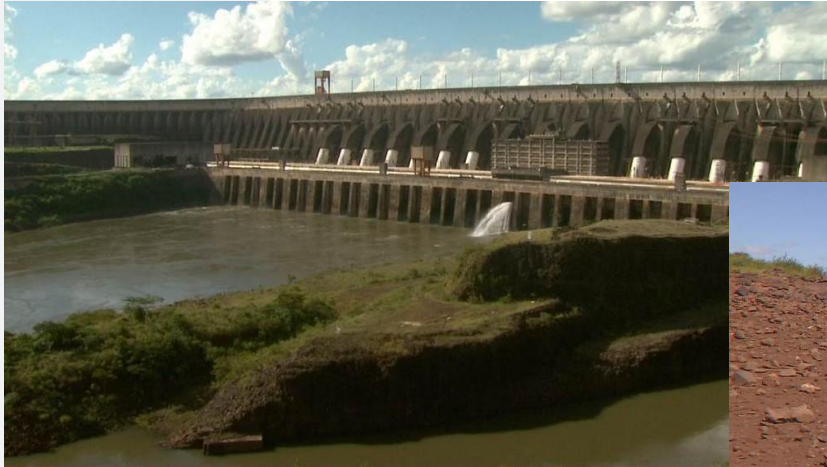
Itaipu Hydro-Electric Power Plant
