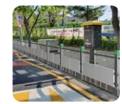
Fine dust absorption wall
