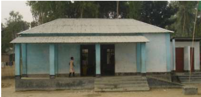
Figure 37: Flood shelter with wheelchair ramp on raised land in Bangladesh. The shelter doubles as a school. Photo: James Pender
