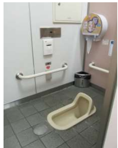
Figure 43: Accessible squat toilet. Photo: Betty Dion
