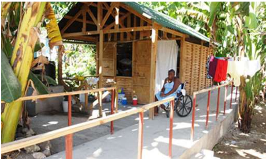
Figure 49: Accessible new housing, along accessible route. Photo: CBM.
