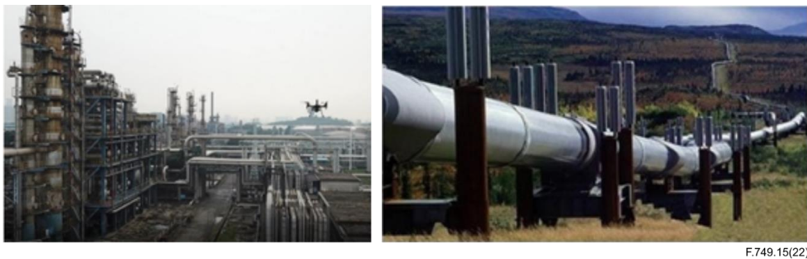
Figure I.3 – Example of oil pipelines and its supporting facilities inspection and examination service
