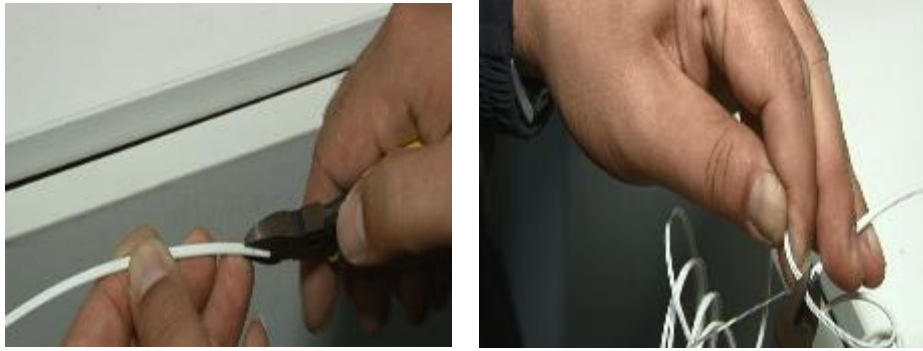
Figure III.11 – Separate the in-home cable from the bow-type drop cable
