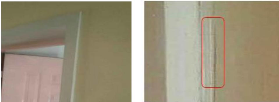
Figure III.12 – Installation of the in-home cable with glue
