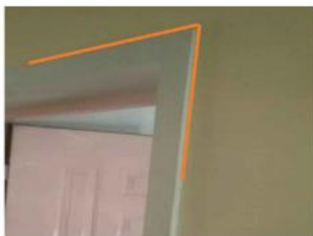
Figure III.8 – Installation of the in-home cable (indicated by orange line)
