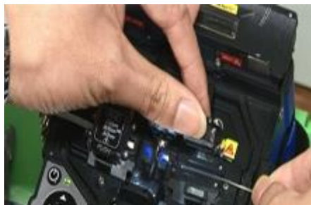
Figure III.7 – Splicing the in-home cable with the drop cable
