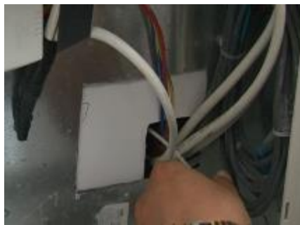
Figure III.6 – Introducing the drop cable to home
