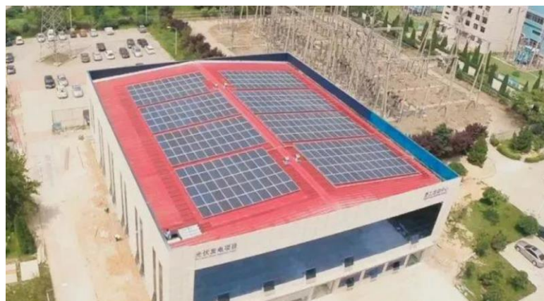
Figure 7 – Example of a roof-top PV near the edge data centre [b-GBWindows]
