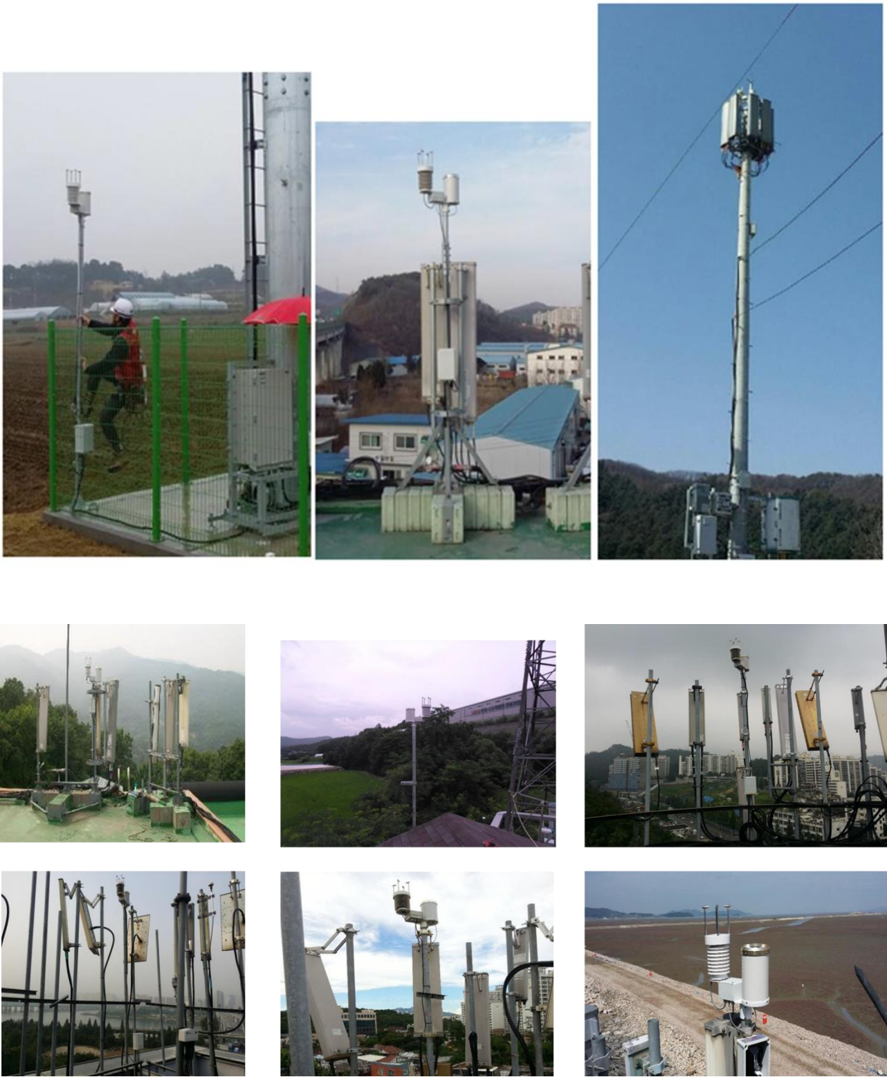
Figure I.4 – Deployment examples of installing environmental sensing system on various ICT sites
