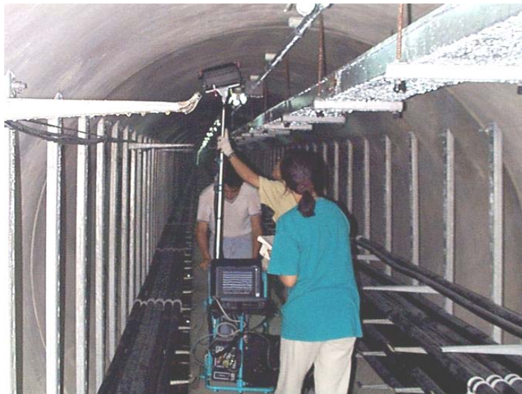
Figure I.4 – Tunnel lining inspection using GPR
