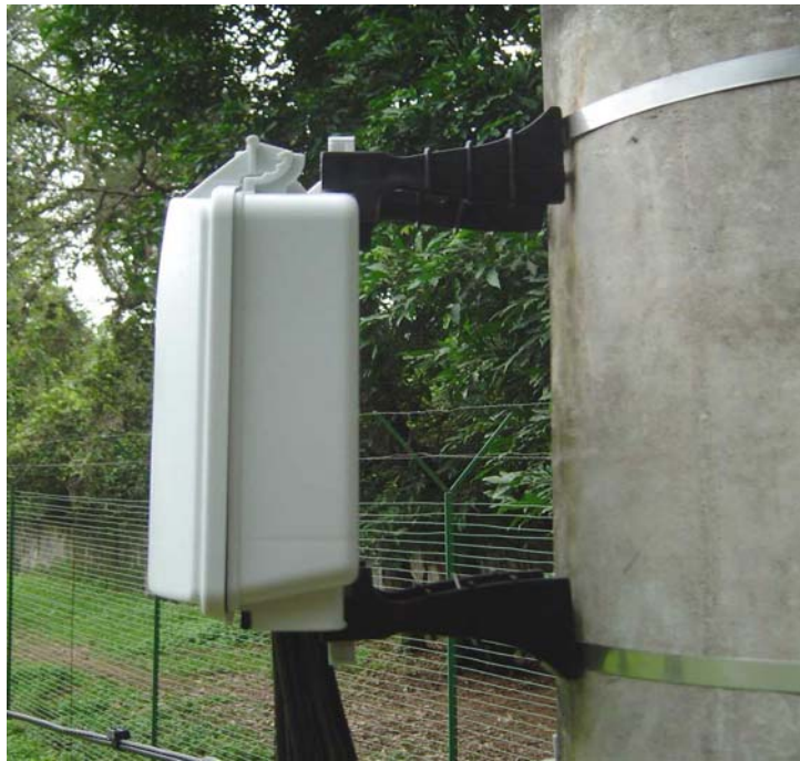
Figure II.8 – Terminal box (TAR)
