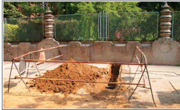
Figure 4 – Digging essay for existing utilities localization
